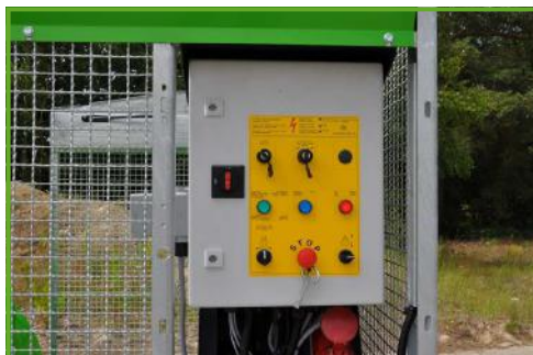
clear control panel
